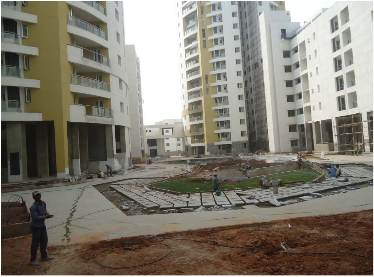
PROGRESS STATUS - CENTRAL COURTYARD
