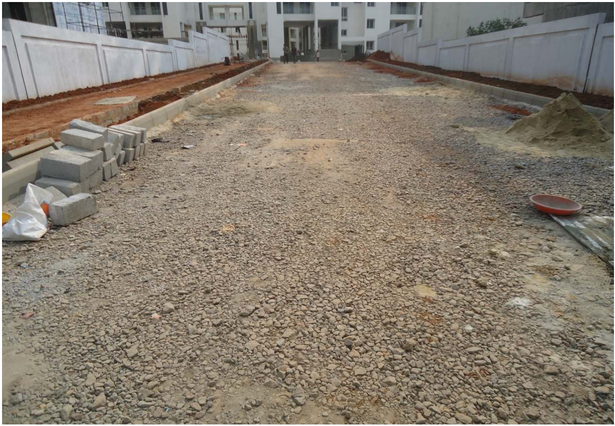
PROGRESS STATUS - MAIN ENTRANCE DRIVEWAY
